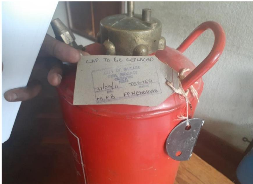
Fig (3) Un-serviced Fire Extinguisher
